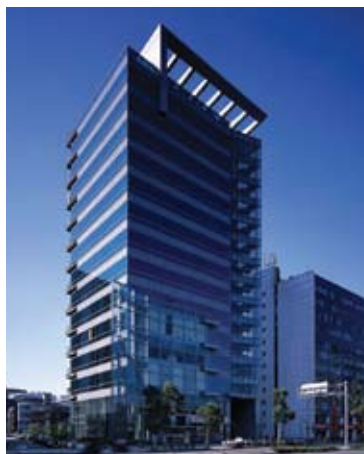
Taiwan Gate Building, an example of one of the newer properties in a sub-market where the average age of the stock is approaching 16 years.
