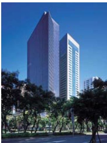
Dun Nan Continental Building (CEC Dunnan), one of the most sought-after properties in Dunhua South.
